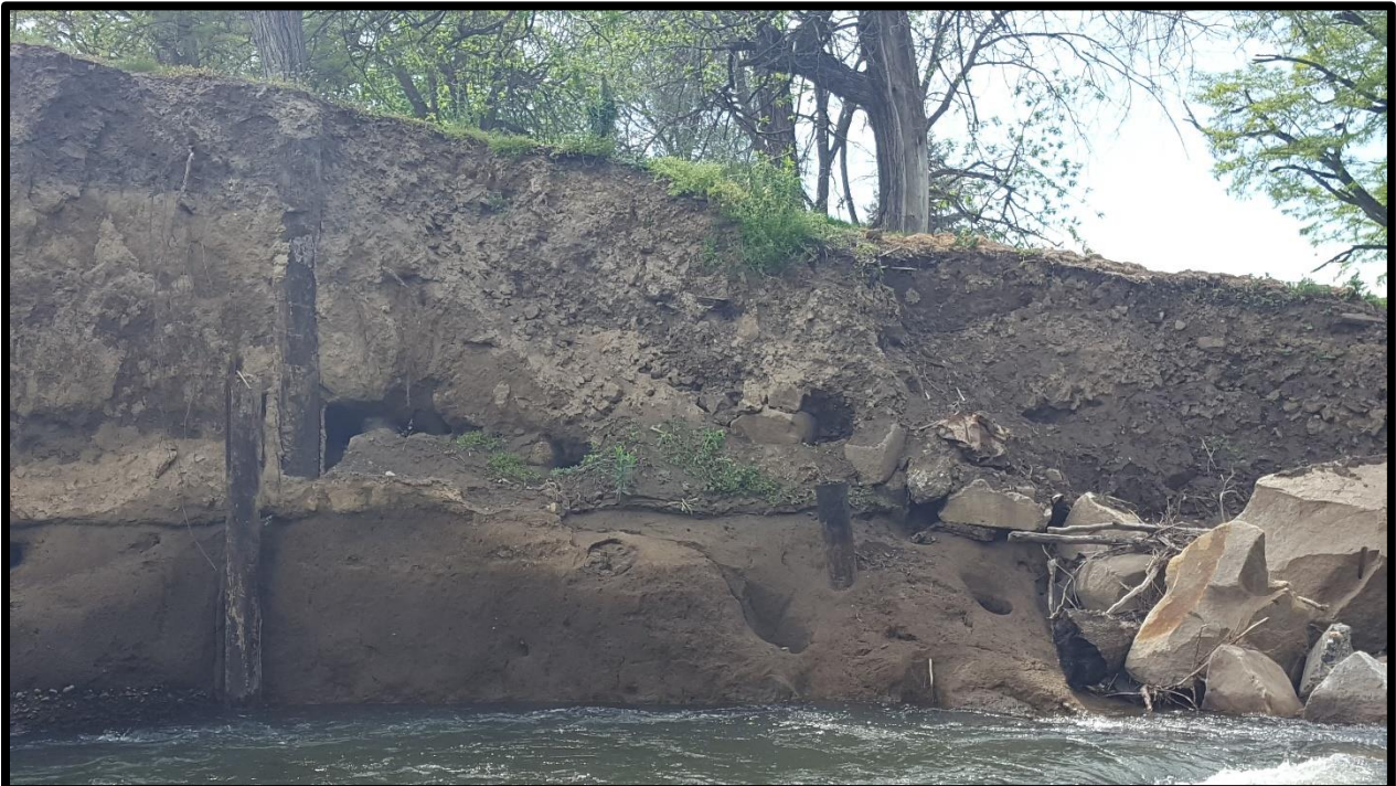
Figure 9. Photo looking south at levee rehabilitation location showing remnant trestle piers, rail bed fill, and levee riprap.
