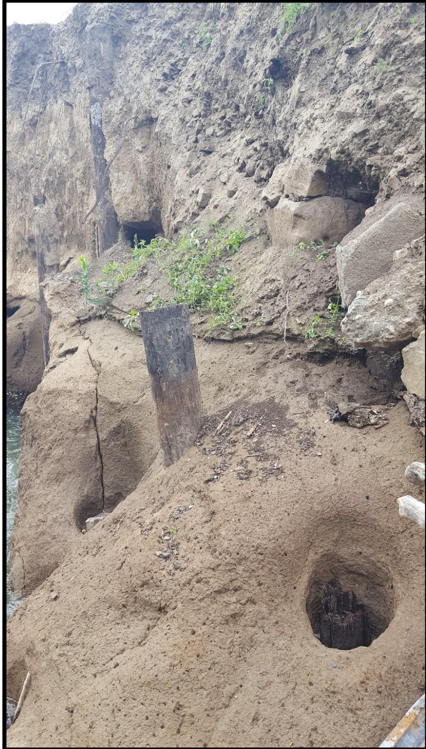
Figure 10. Photo looking upstream along bluff showing remnant trestle piers and rail bed fill (upper right).
