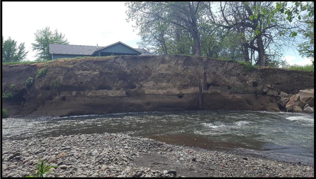
Figure 8. Photo looking south at levee rehabilitation location showing remnant trestle piers and modern house within railroad right-of-way.
