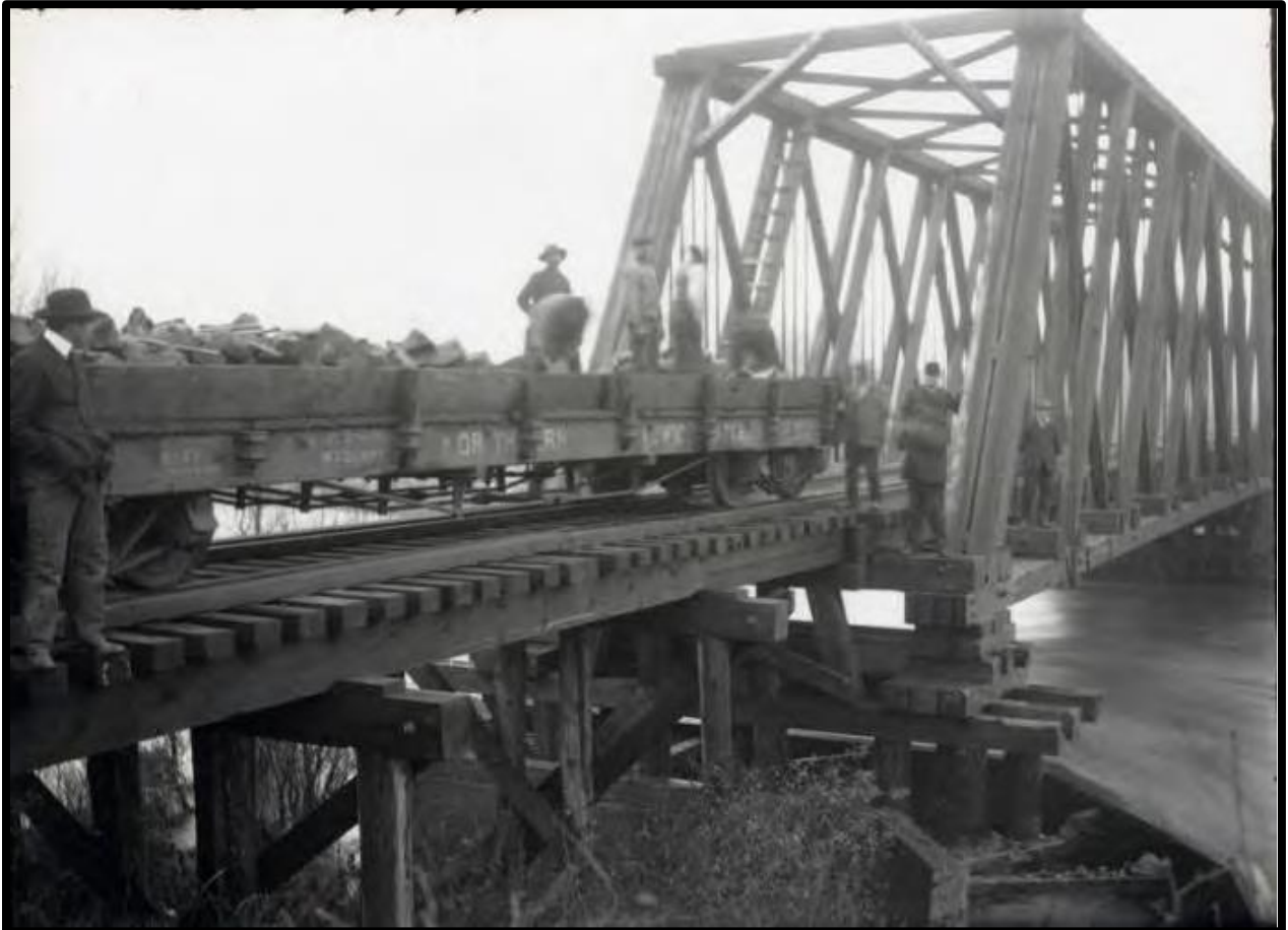
Figure 6. Historic photo of railroad trestle over the Touchet River at River Mile 44.5 showing foundation piers. Photo courtesy of the Waitsburg Historical Society and Tom and Anita Baker (from Amonette 2009).
